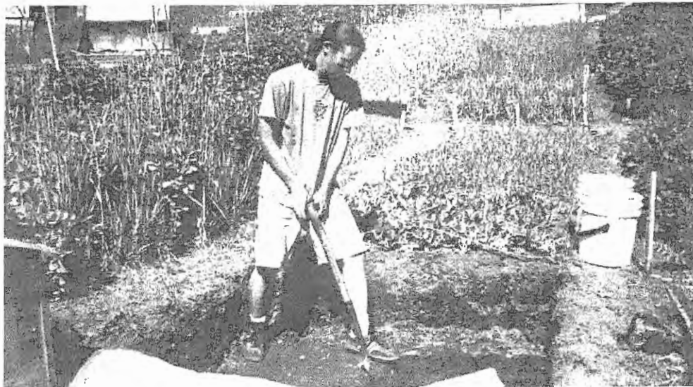
Dan digging out the lower 12 inches of soil for the new gopher cage
